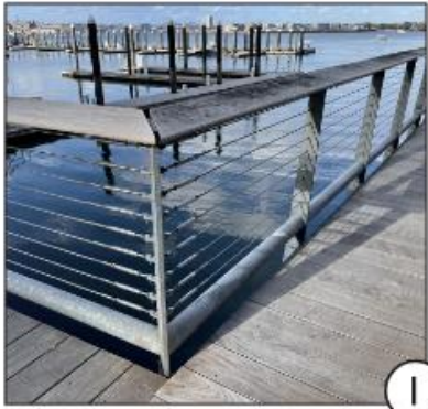
WOOD AND CABLE
