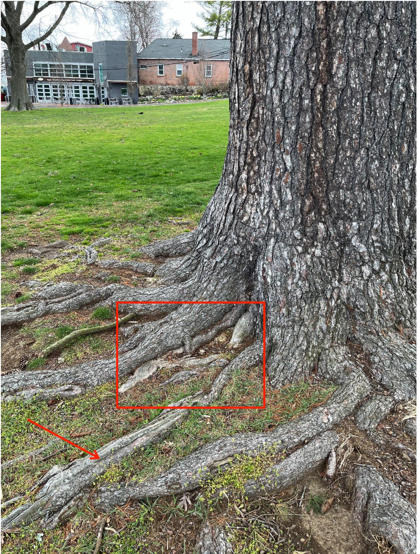
Potograph #13: Tree #2 Surface roots with mechanical damage.
